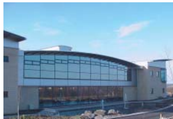
Factory constructed by Scottish Borders Council for Plexus at Pinnaclehill, Kelso
