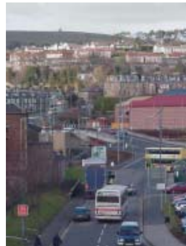
The Hawick traffic relief scheme has resulted in major benefits to the main shopping areas in the town.
