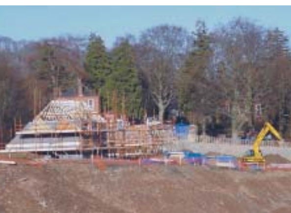
New housing under construction at Abbotsford Road, Galashiels
