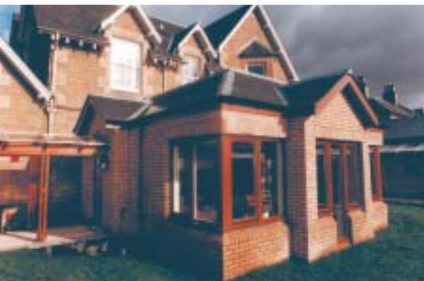
Special needs housing, Melrose
