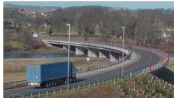
Hunter Bridge, Kelso. Completion of the outer distributor road and new bridge in 1998 alleviated traffic congestion in the town centre and improved journey times.
